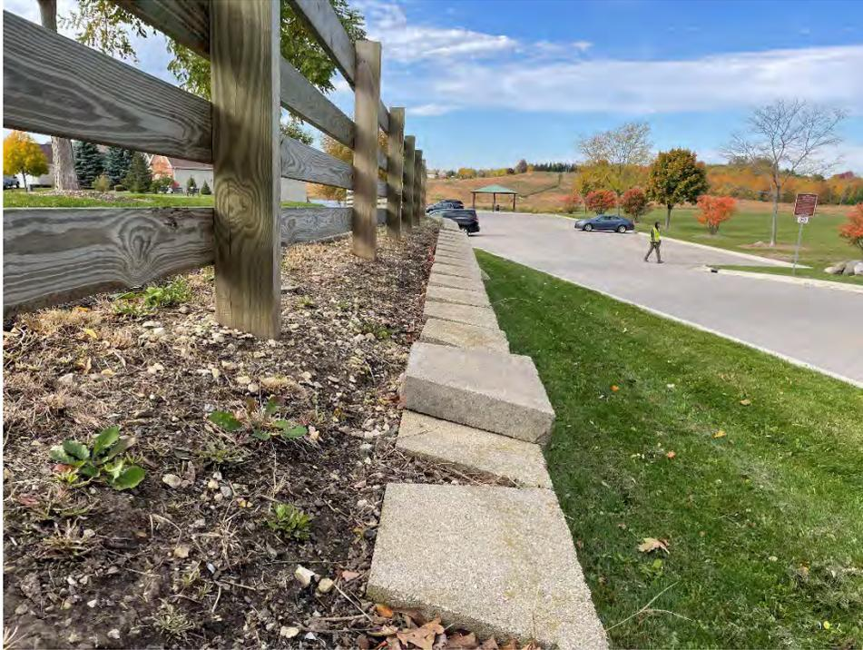
Top of Wall Looking West – Wall is Leaning Forward - Note that the Standard Batter for an Anchor Diamond Wall is 10.6° Back. Front Face Angle Measured Up to Approximately 89° (Up to 10° Forward)
