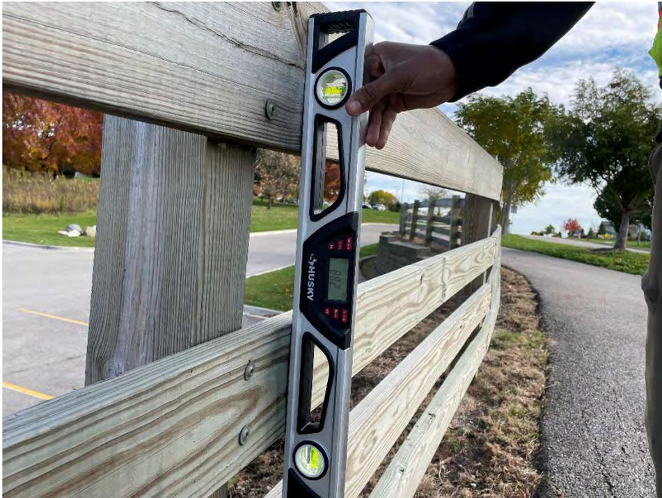
Wooden Railing Leaning – 88.2° at 60' from West End of Wall, 84.1° at 80' from West End of Wall
