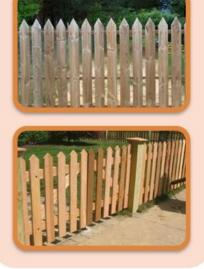
Semi-Open Fence (ex. board-on-board, shadowbox, etc.)
