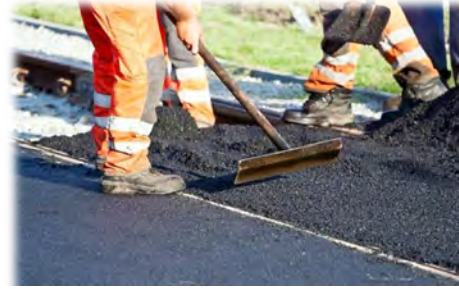
The MFT Fund assigns resources for repairing and resurfacing Village streets for improved travel
