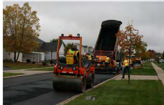
Resurfacing work performed on a residential street in Algonquin
