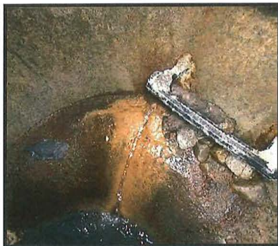
Leak at Wall
