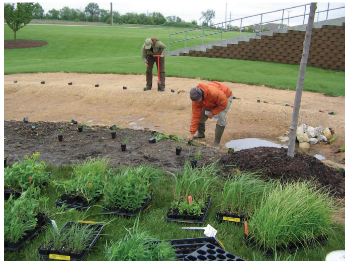
Rain Garden planting at water treatment plant on Academic Drive.
