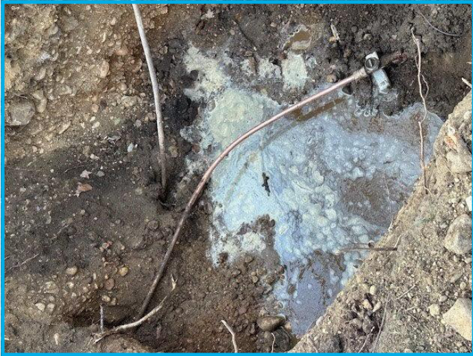
Replacing Lead Service Line With Copper Service Line
