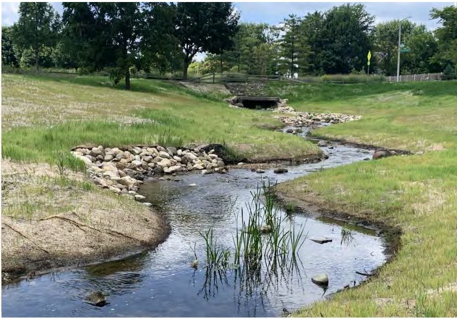
MEANDER CHANNEL SECTION WITH EXTENDED STONE TOE PROTECTION & BENCH (APEX OF MEANDER) NO SCALE
