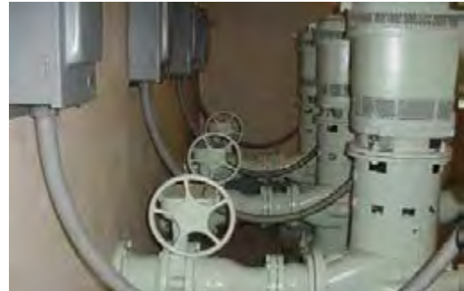
High Service Pumps at Water Treatment Plant No.1 to receive VFDs with PZ2 Improvements.
